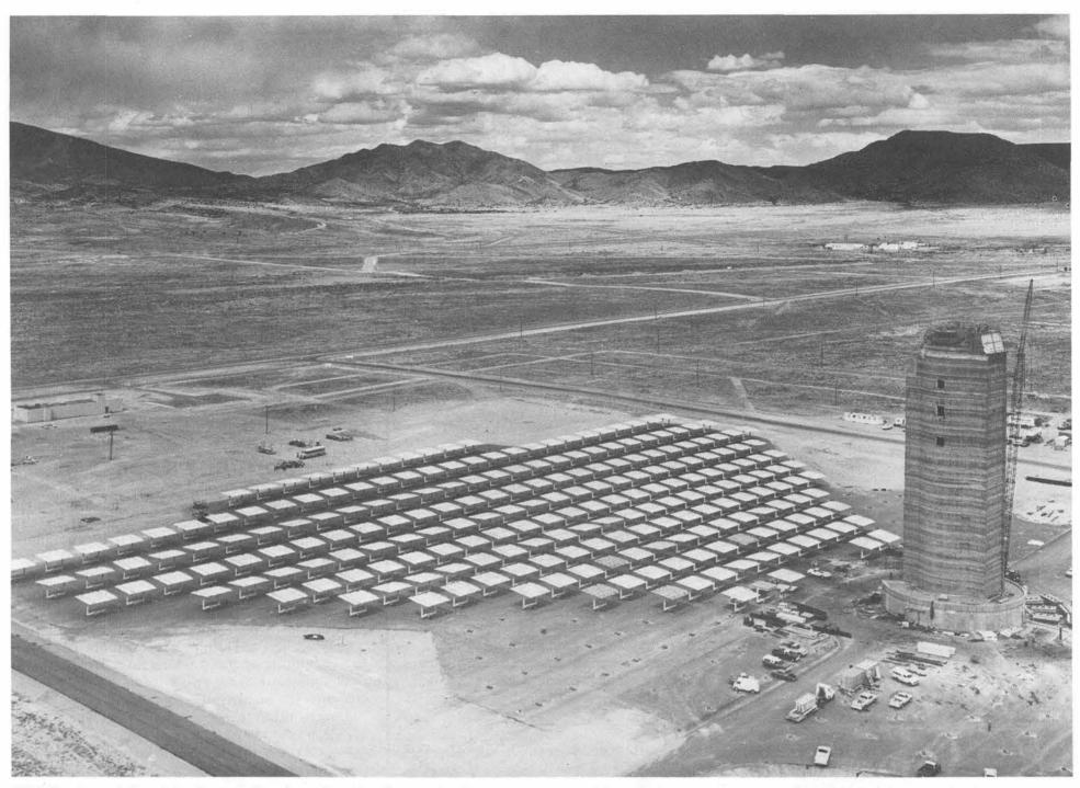
AERIAL view of Sandia's Central Receiver Test Facility — the Power Tower — was taken shortly before facility was completed. Experimental boilers have since been installed and testing is underway. An unusual night-time experiment was recently completed here, using the array of mirrors to focus radiation from celestial and atmospheric events onto detectors as a possible means of detecting the explosion of black holes in space. Story on page 7.
